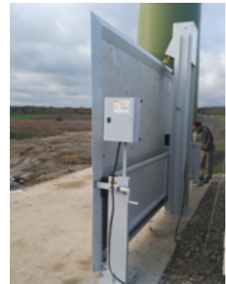
Box for protecting the control pendant in the version with electric chain hoist.
