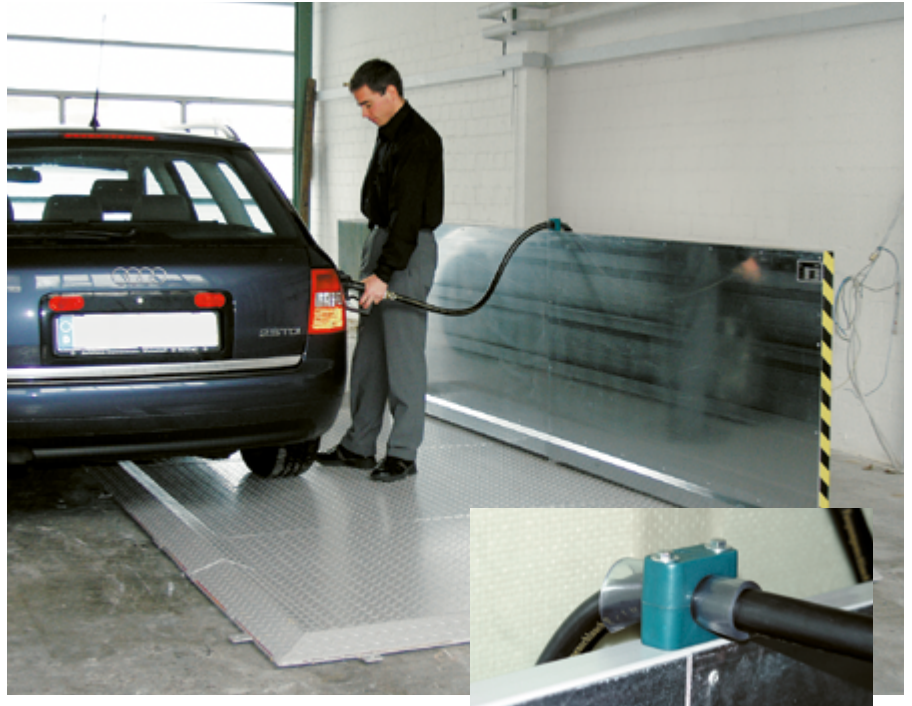
Compact fuel dispensing area
