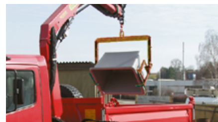
Tipping the grit out onto a truck platform (shown with 700L grit bin)
